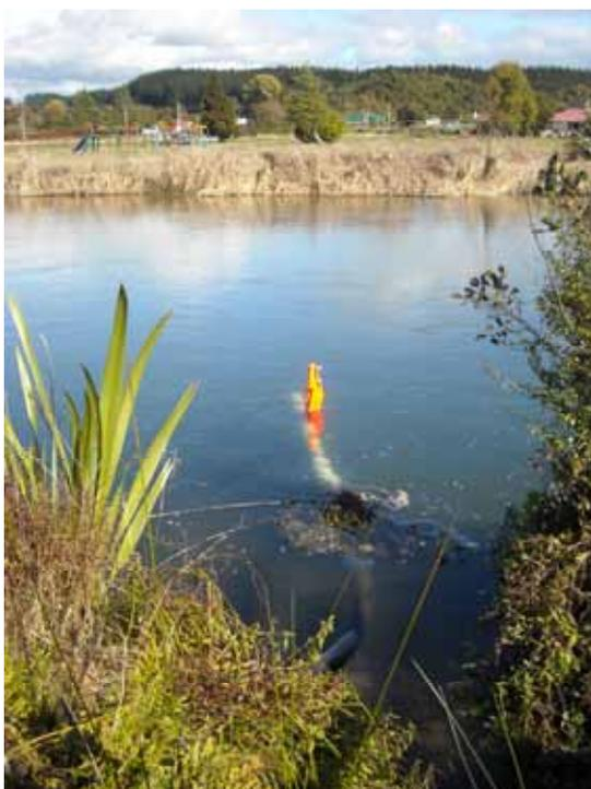
*Figure 3 Orange safety flagged water intake on the Ōhau channel.*
