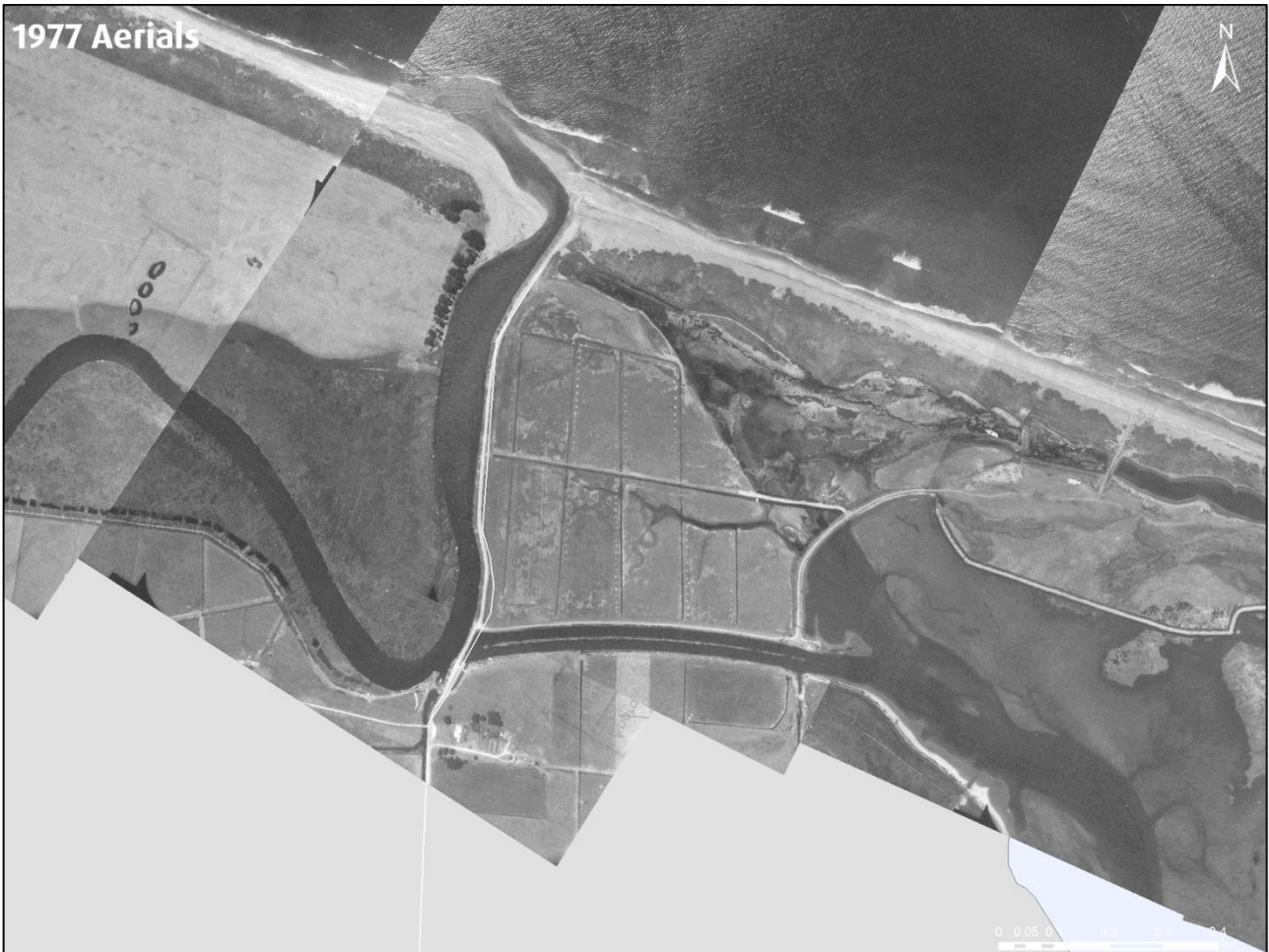
Figure 3: Aerial photograph of Te Tumu area in 1977. Note significant loss of wetland extent, and additional stop-banking. Northwest of Papahikahawai Island macro-algal growth is visible.
