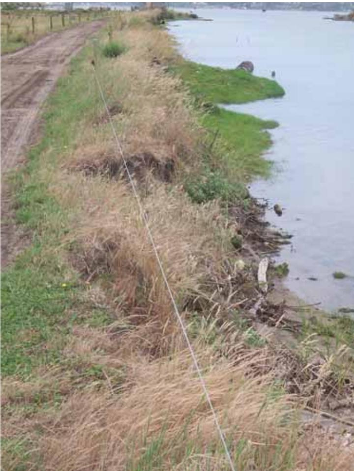
Photo 4 Erosion extending beyond fenceline
