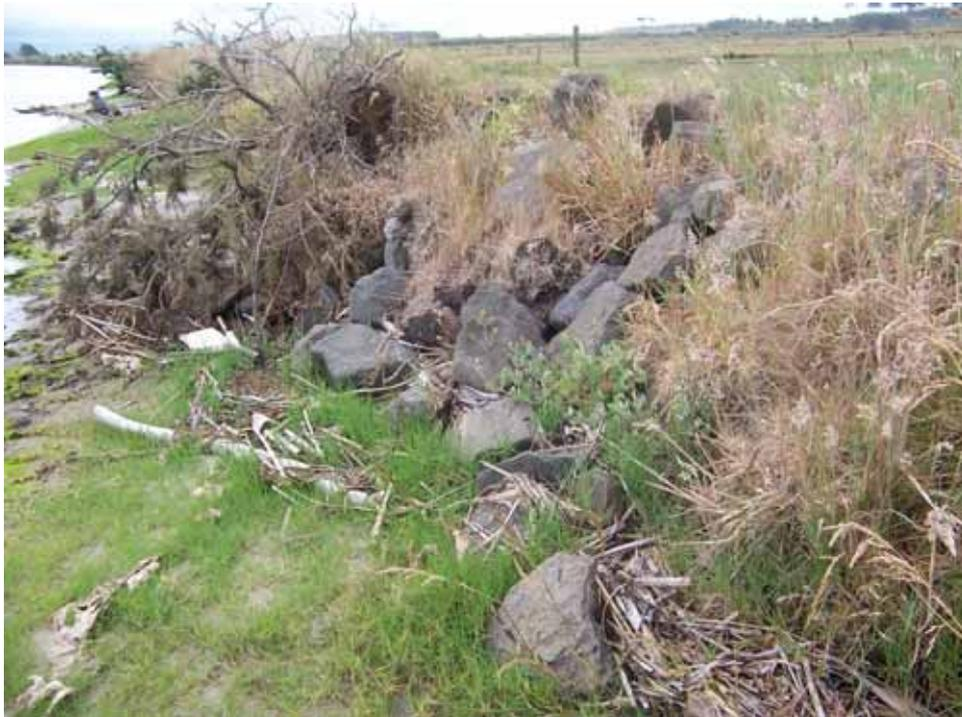
Photo 5 Isolated older rock protection. Grass-like vegetation establishing on beach. Note debris line indicating recent highwater mark
