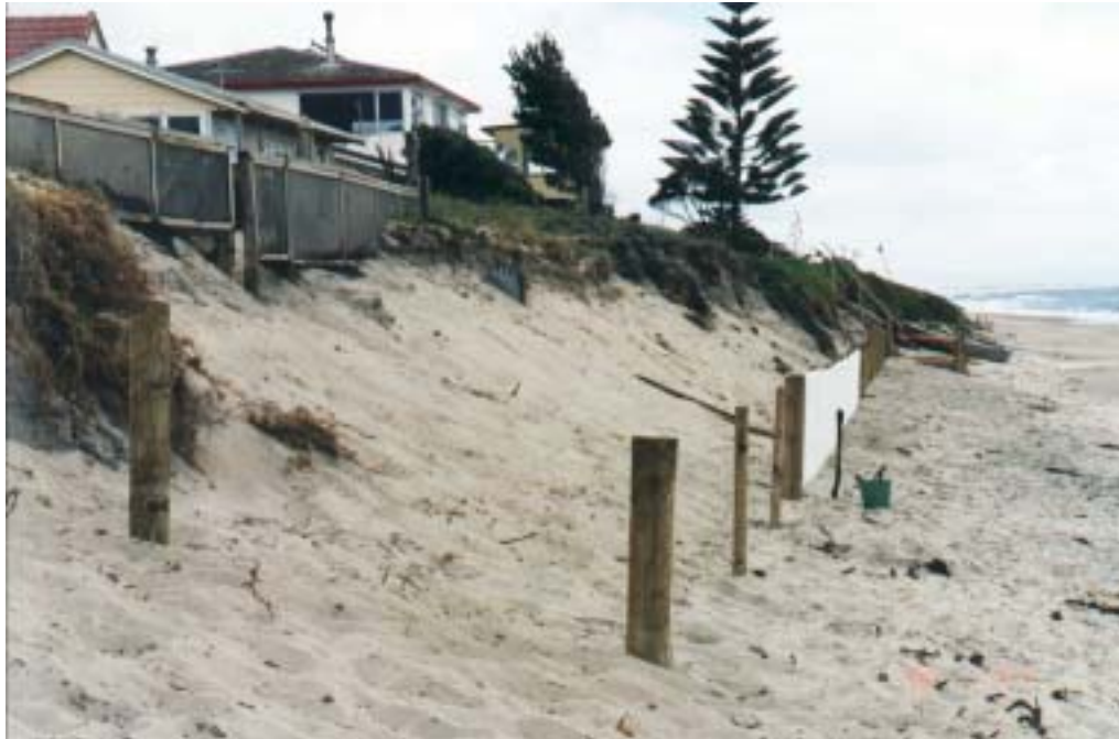
Coastal protection works at the toe of the foredune at Papamoa - 1997
