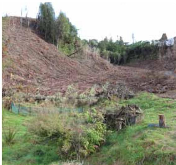
*Silt fence as final perimeter control below forestry operations.*
