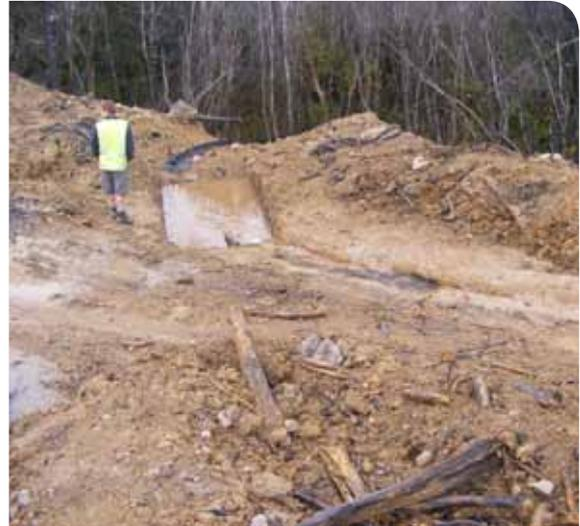
*Sediment trap has been installed in stable ground. Discharge is through a flume over the batter slope*
