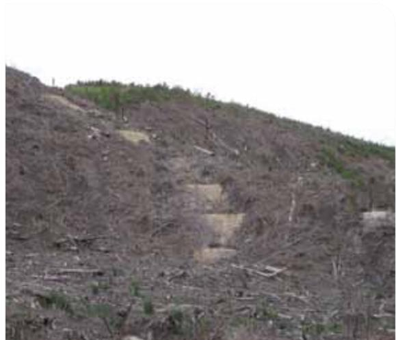
*Water bars installed in decommissioned haul track on pumice soils.*
