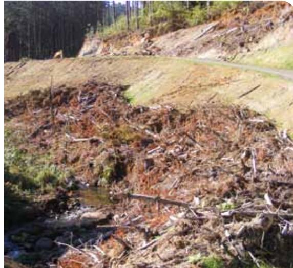
*Combination of hydroseeding, grassing and slash to stabilise ground surface and help filter any sediment before reaching stream channel*
