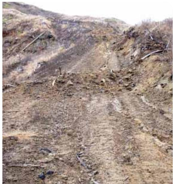
*Cut off installed on haul track diverting water onto stable outfall area.*
