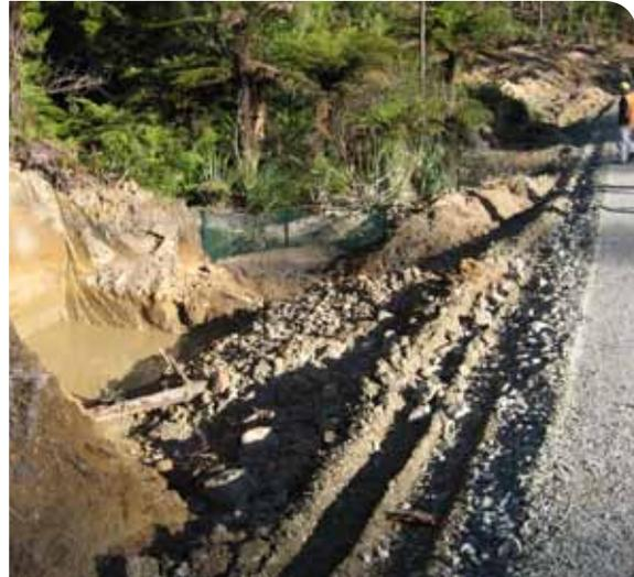
*Soak hole plus silt fence where the discharge point is close to a stream*
