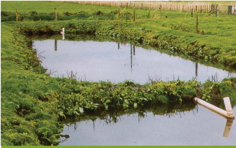
Two pond system with T-baffle pipes (photo courtesy of New Zealand Dairy Research Institute)
